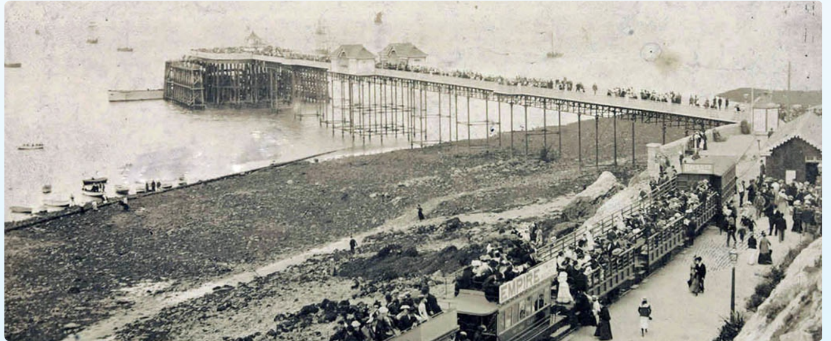
The Mumbles Pier
